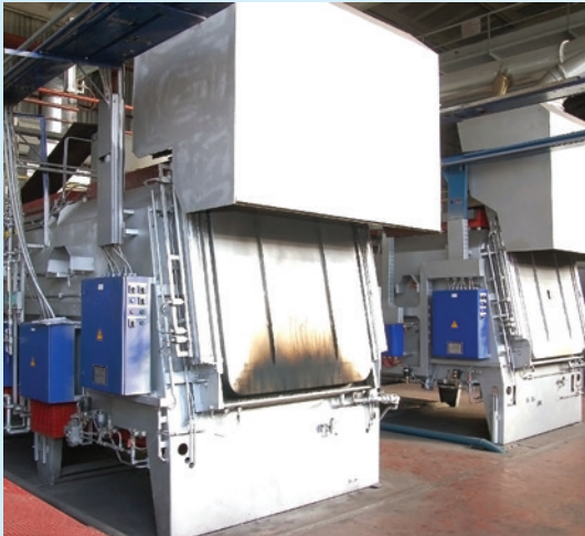
Medium scale multi-process multi-PID loop manufacturing lines
